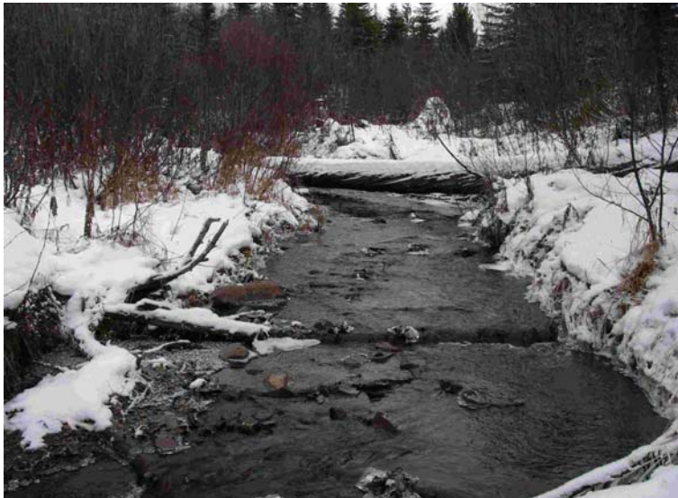
Photo 21 – Whiskey Br. area, trib. with 18" & 24" culverts.
