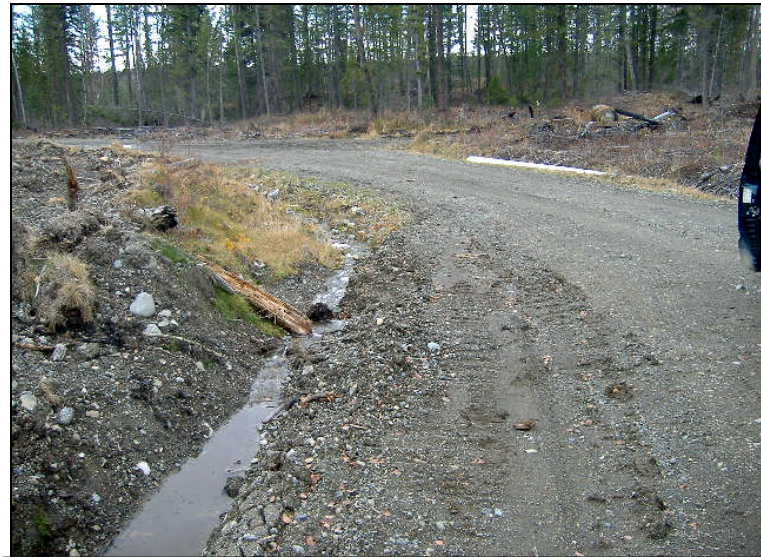
Photo 30 – Sucker Creek area, typical new road.
