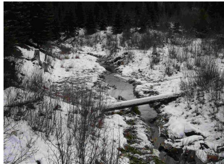
Photo 20 – Whiskey Bridge area, trib. with 36" culvert.
