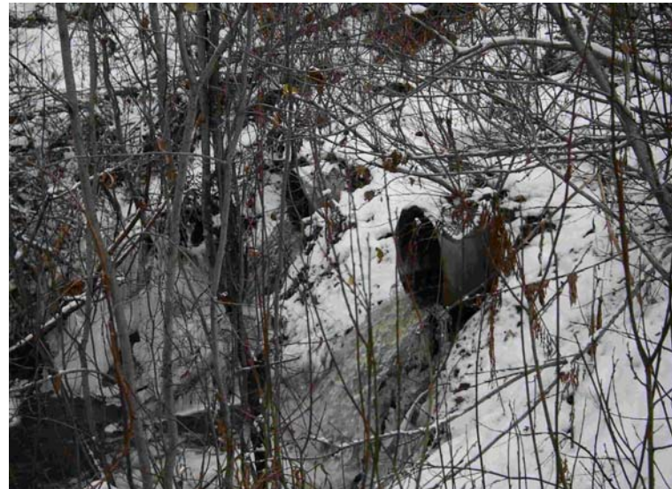
Photo 22 – 18" and 24" culverts outlets.
