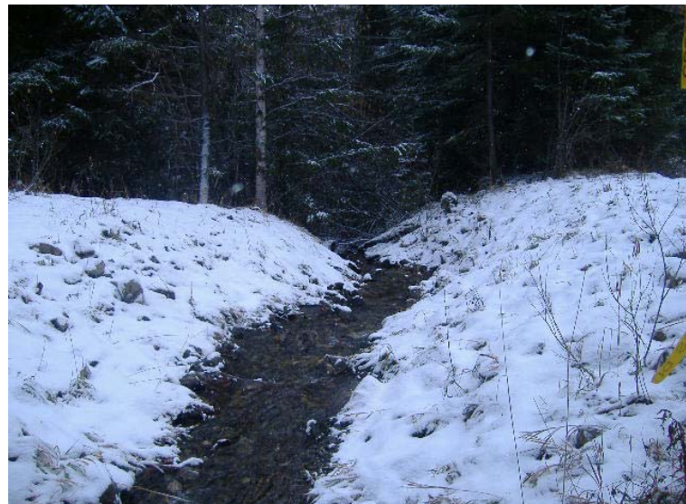
Photo 24 – Deactivated spur road on 141 km tributary.
